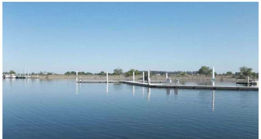
The City of Richland is using a $49,000 Boating Infrastructure Grant to provide power to the Columbia Point Marina Park boat docks.
