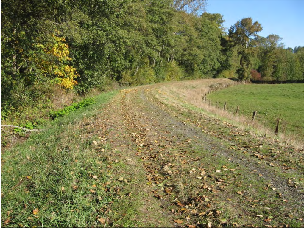
Photo of levee on property, looking north
