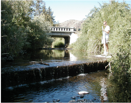
North Yakima Conserv Dist; Restoring Fish Passage on Cowiche Creek (#16-1753) Attachment #257849, P7310029
