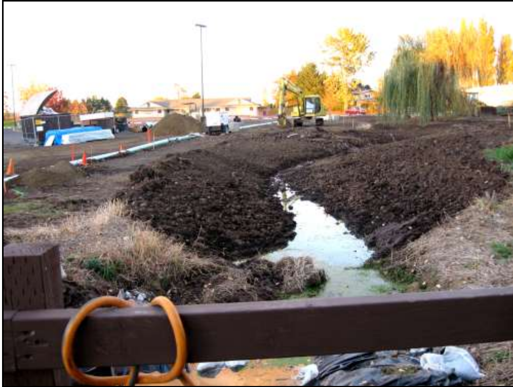
Figure 16. Titus Creek channel reconfiguration at Walla Walla Community College Campus
