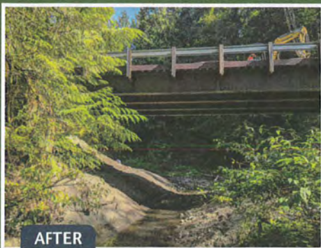
A new 65-foot bridge replaces the undersized culverts on Swede Creek allowing fish to migrate upstream and access high quality habitat.
