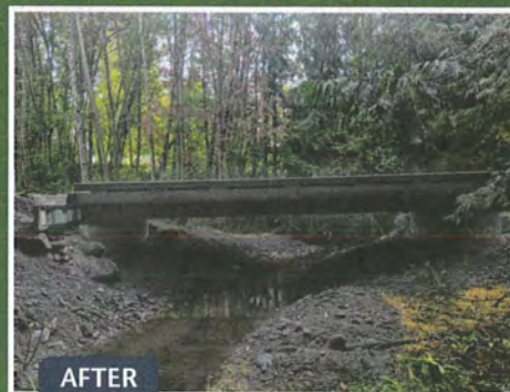
A new 30-foot bridge replaces the undersized culverts on Carpenter Creek allowing fish to migrate upstream and access high quality habitat.
