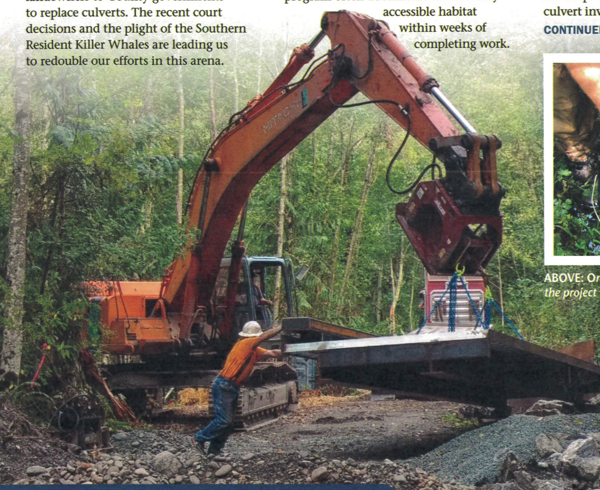
Installation of a new bridge on Carpenter Creek removes a fish passage barrier
