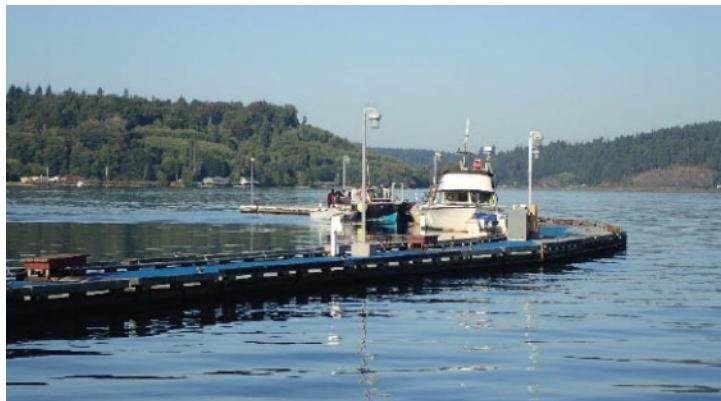
Port of Bremerton, Port Orchard Marina Breakwater #20-1855
