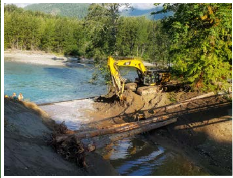
Removing the "plug" to reconnect Pressentin Slough to the Skagit River.
