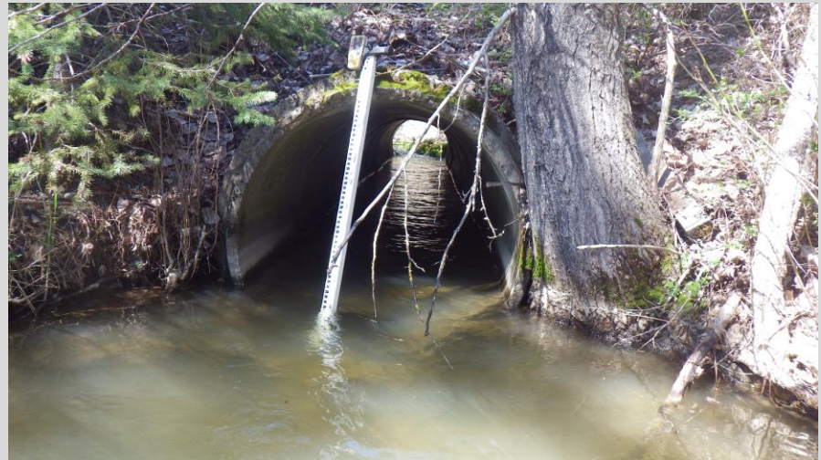
Crystal Creek. Spring 2022. Completing downstream barrier assessments with Trout Unlimited.
