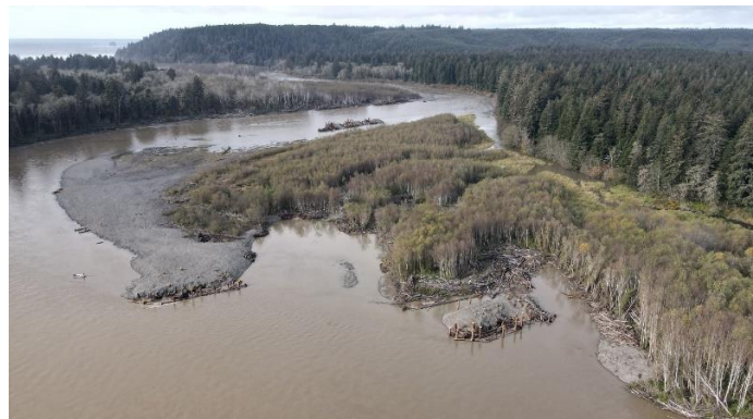
Completed log jam installations done in Reach 3 Photo Courtesy of the Quileute Tribe
