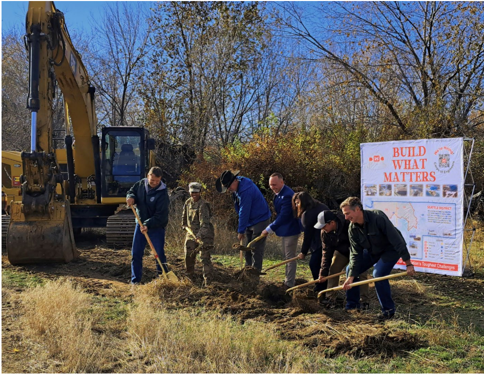
Local, State, Federal & Tribal Partners at the Groundbreaking.
