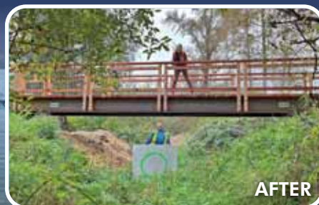
Showing the size of one of the removed culverts with the newly completed bridge that allows salmon to migrate upstream and downstream while also providing park visitors better trail access.
