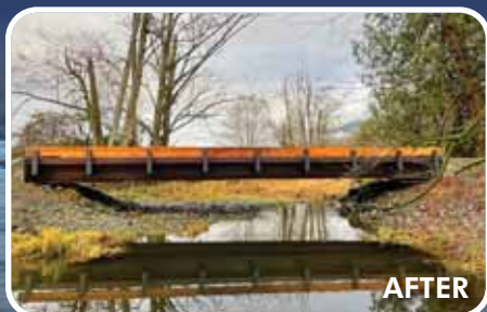
New bridge on Lower Day Slough allows unimpeded access to adult and juvenile salmon.
