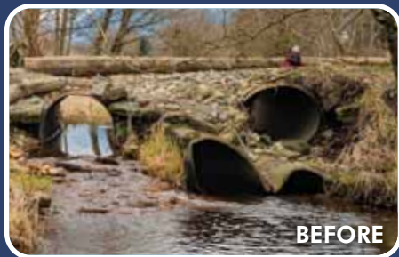
Culverts on Lower Day Slough blocking salmon migration to important off channel habitat.
