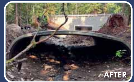
New large culvert reestablishes fish passage on Thompson Creek for salmon and steelhead.
