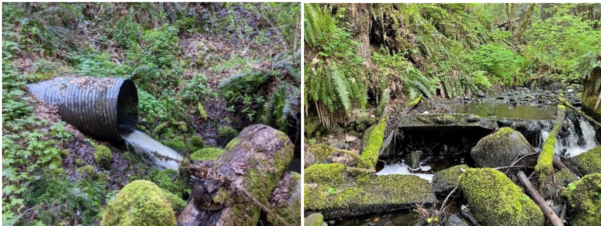
Brighton Creek Culvert Photo credit: S. Motsenbocker
