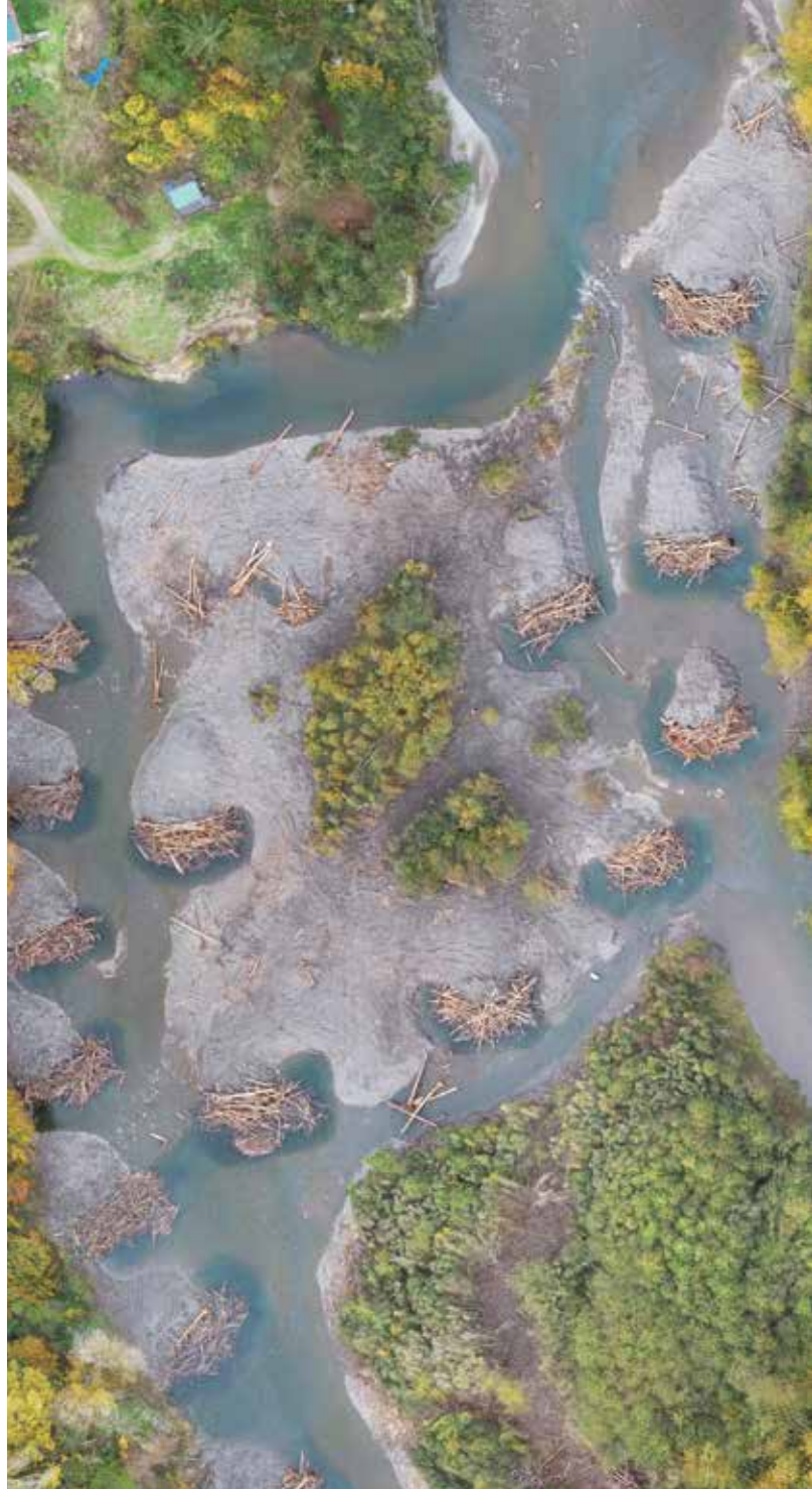
Engineered logjams were installed in the Elwha River in summer 2024 to enhance salmon habitat. Natural Systems Design
