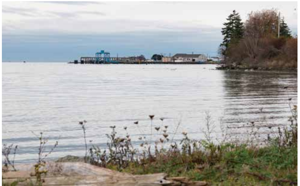
The Lummi Island ferry dock and neighboring piers are seen from across Fisherman's Cove along the Lummi Reservation. Lummi Nation will soon replace its pier and docking infrastructure adjacent to the ferry dock to better support its tribal fishing fleet. Kimberly Cauvel
