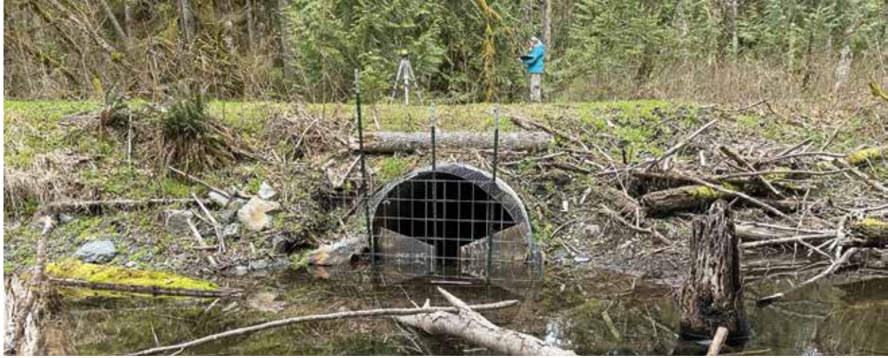
Skagit River System Cooperative restoration ecologist Sue Madsen takes notes at an undersized, debris-impacted culvert on a Forest Service road crossing over False All Creek.
