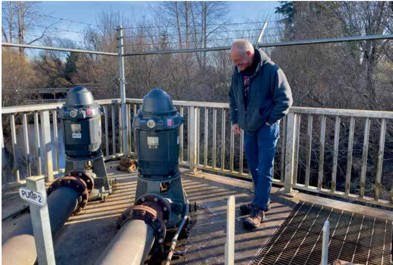
Above: Puyallup Tribe of Indians fisheries enhancement chief Blake Smith inspects vertical turbine pumps, a new addition to the tribe's Clarks Creek Hatchery. Trevor Pyle
